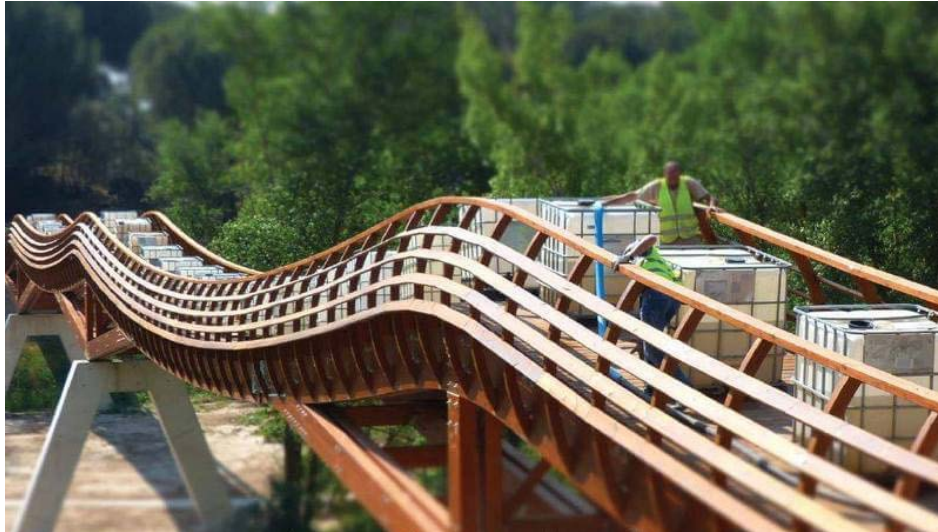
Figure 1. Loading test in a timber footbridge.
