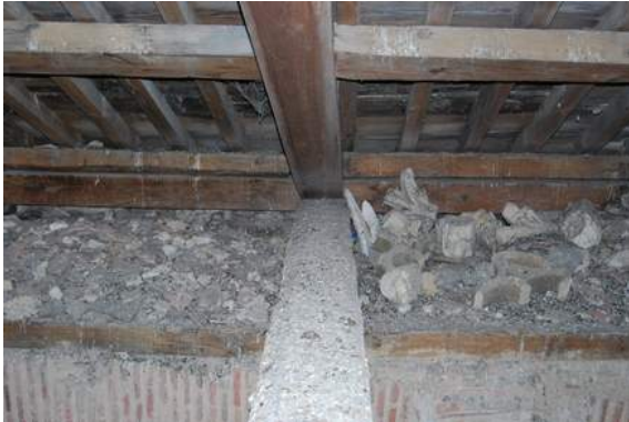
Figure 9. Waning on rafter tie.
