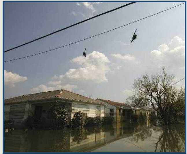
Figure 1. — Flooding in the aftermath of Hurricane Katrina, which caused severe damage to structures in New Orleans.
