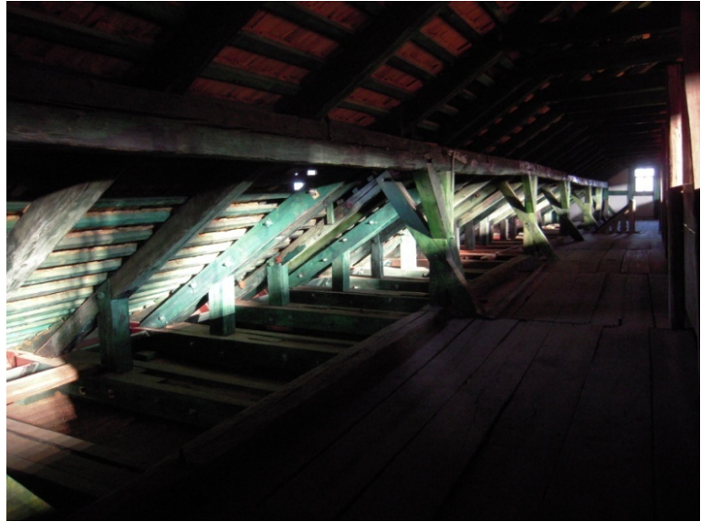
Protestant Workstoffbau church of Javor Strengthening of the structural system (left) and the rafters of the roof, following the trend "timber to timber".
