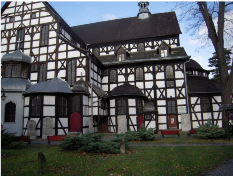
The Protestant Timber Church of Swidnicza built with the Fachwerkbau system
