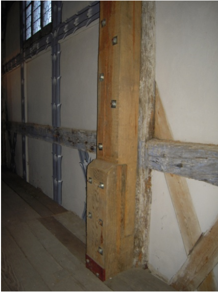
Protestant Workstoffbau church of Javor Strengthening of the structural system (left) and the rafters of the roof, following the trend "timber to timber".
