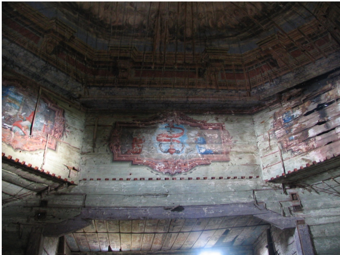
Pictures of the interior of the Church and of the material and structural failure of the dome and its supports
