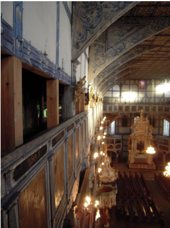
Protestant timber Church of Javor, Poland, affected with soil settlements (the effects are visible at the beginning of the right wall (left side in the second picture), instability).
