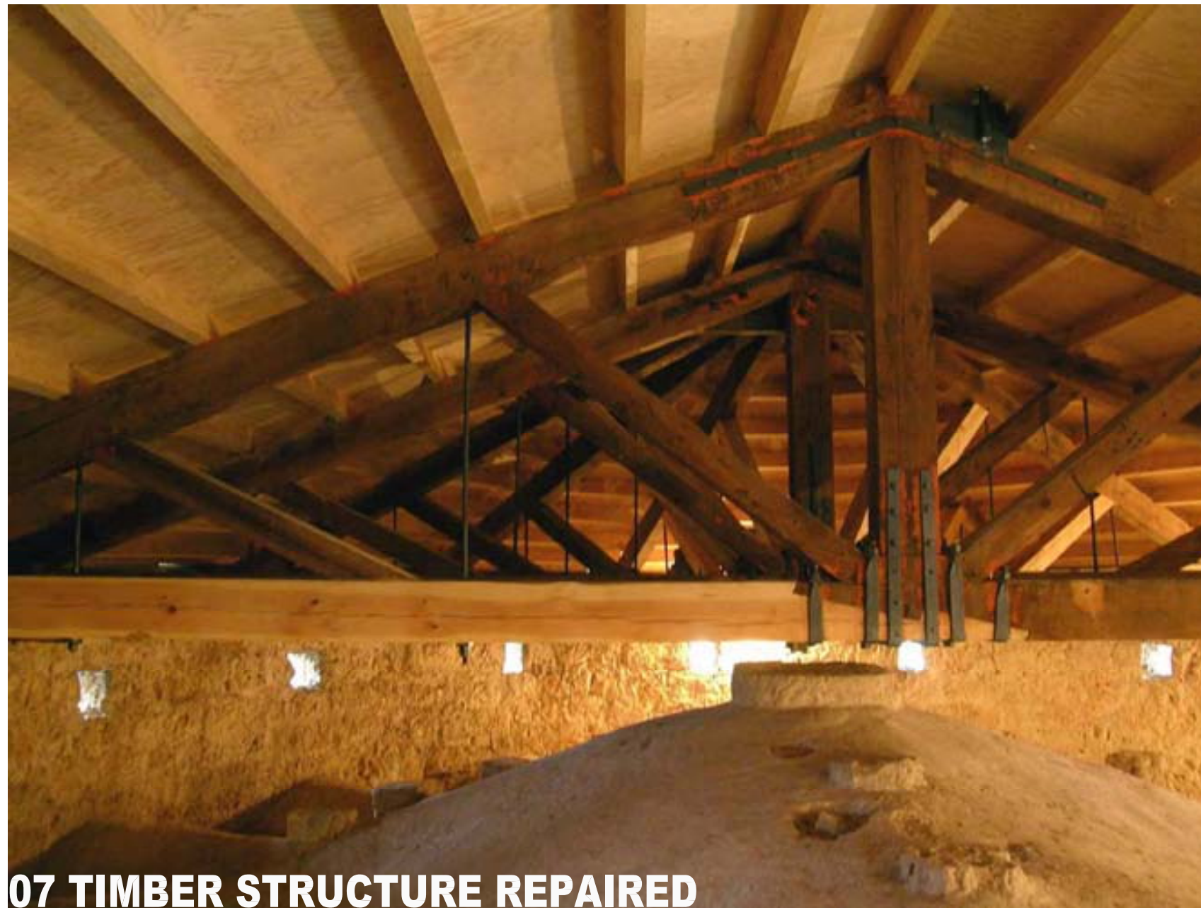
07 TIMBER STRUCTURE REPAIRED
