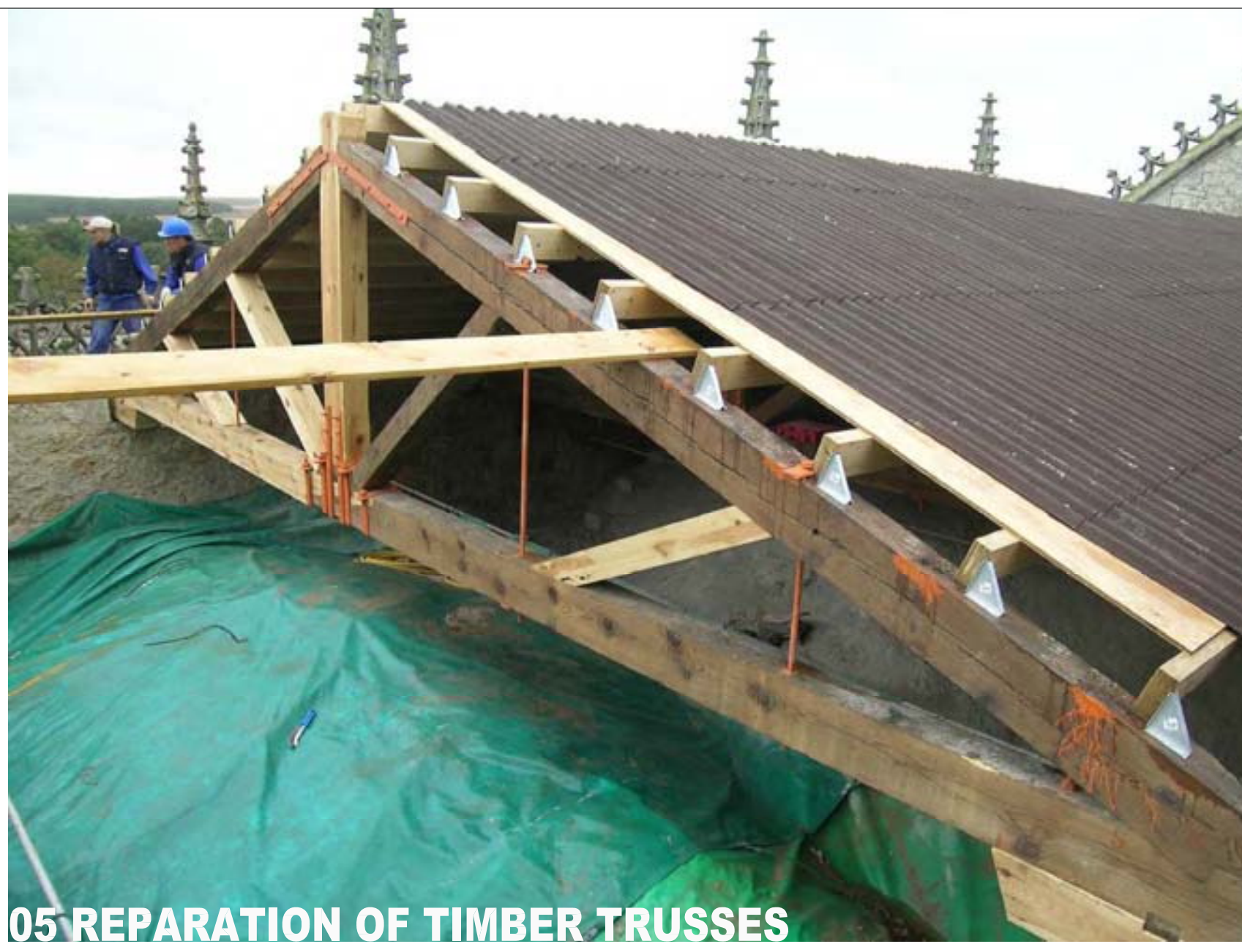
05 REPAIRATION OF TIMBER TRUSSES
