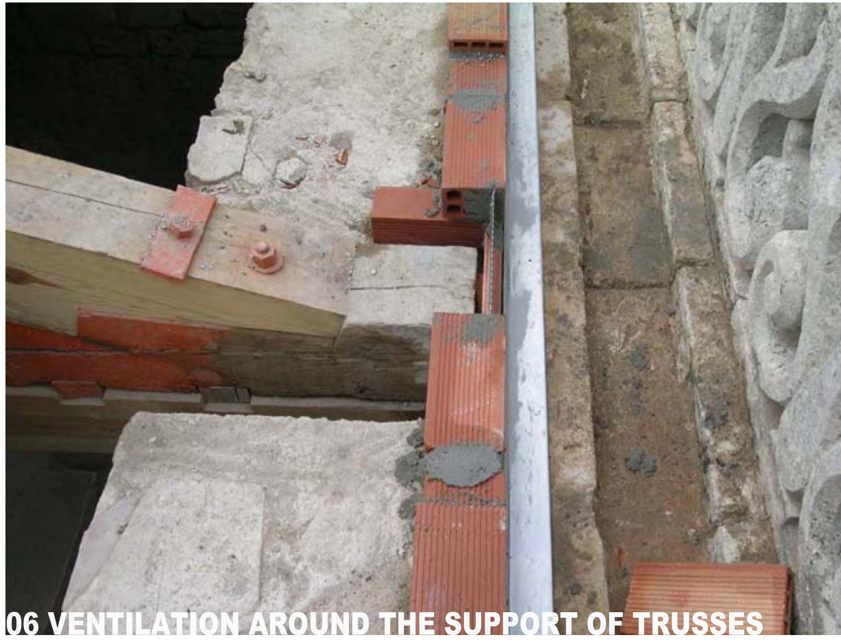
06 VENTILATION AROUND THE SUPPORT OF TRUSSES
